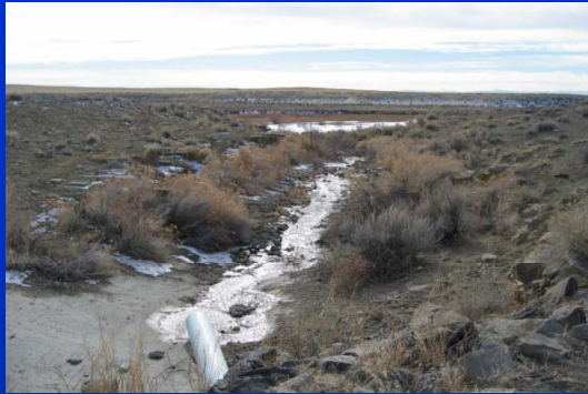
Discharge point from the Shoshoni wastewater treatment plant which discharges to Poison Creek
